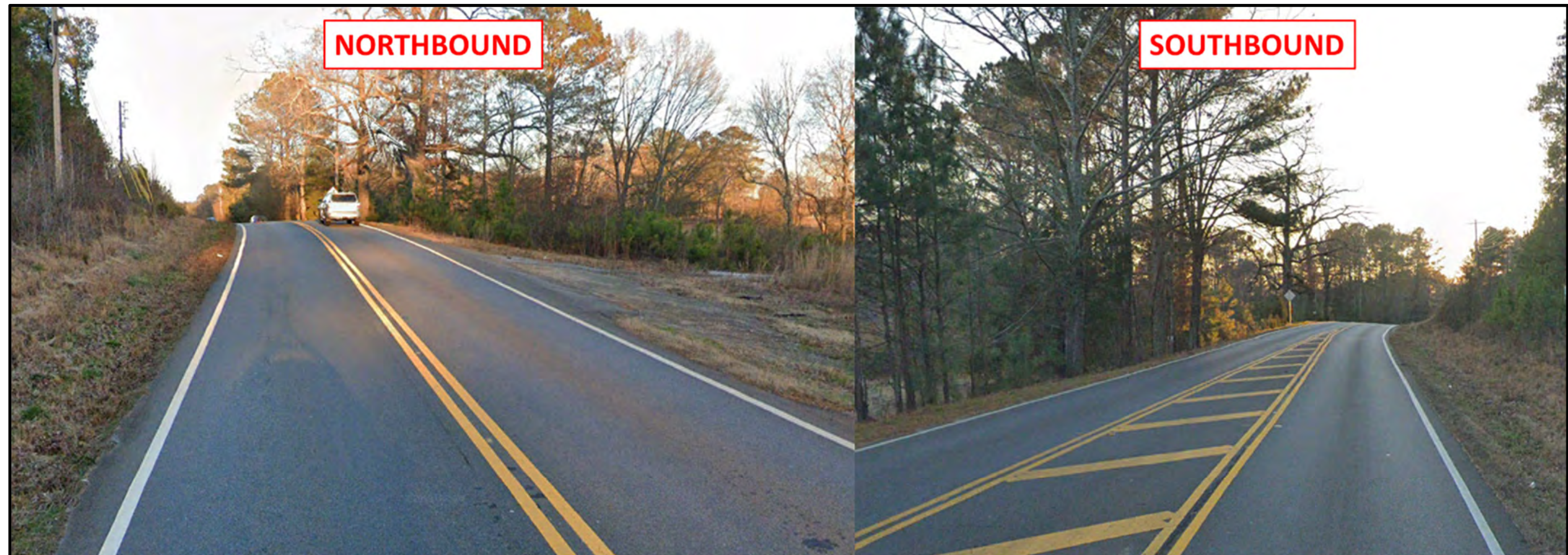
Figure 9: VERTICAL CURVE SOUTH OF STEELS BRIDGE ROAD
