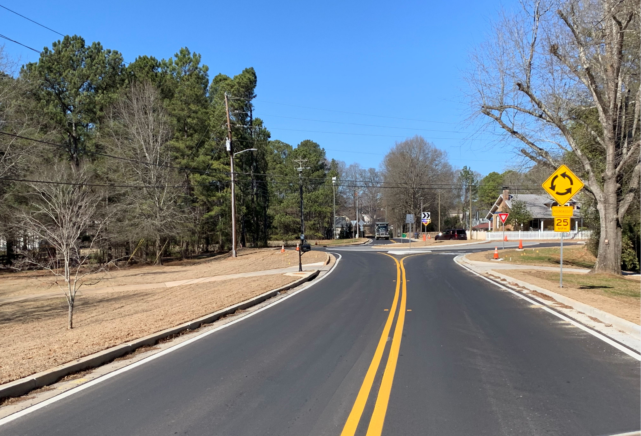
WILEY BRIDGE ROAD AT COX ROAD ROUNDABOUT PROJECT
