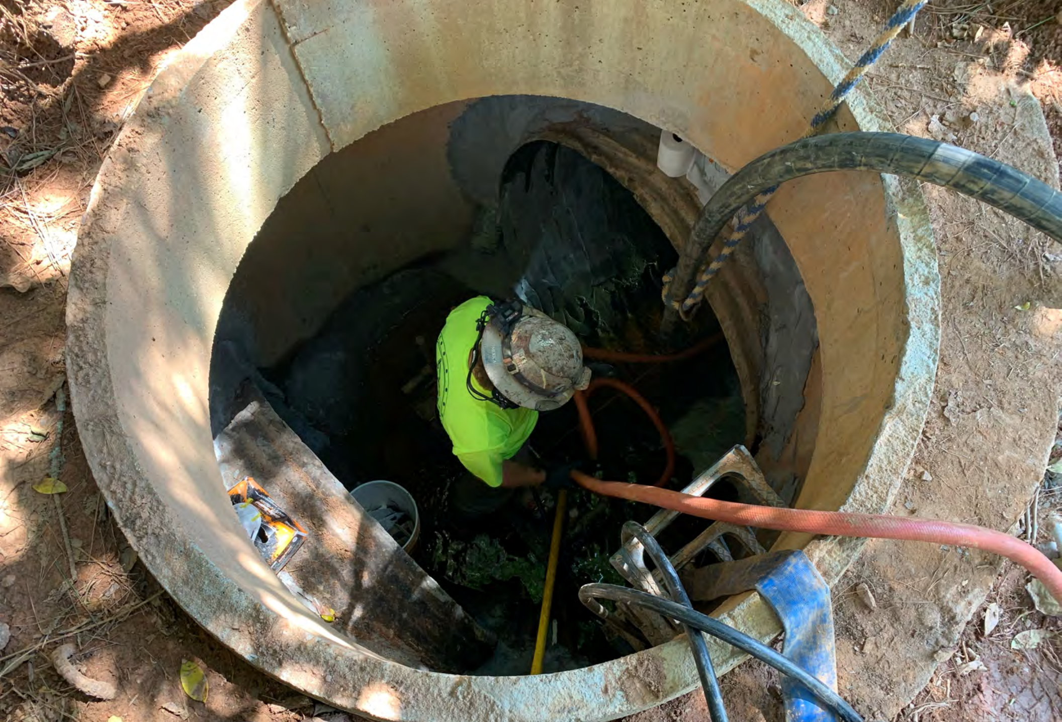
ETOWAH VALLEY ESTATES DRAINAGE IMPROVEMENTS
