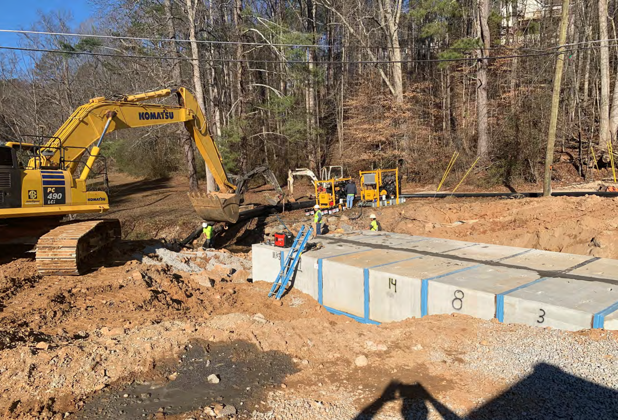
SHOAL CREEK ROAD BOX CULVERT REPLACEMENT
