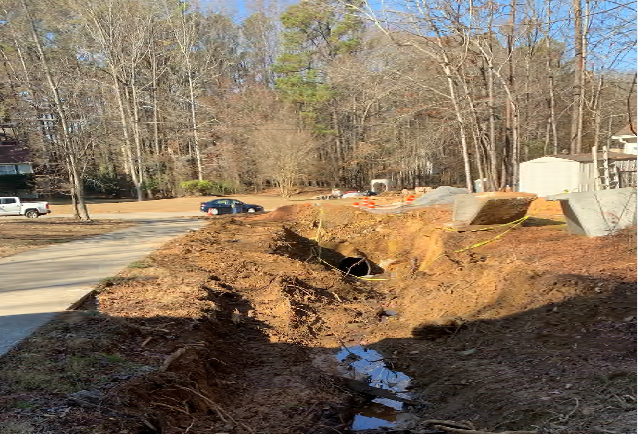
NORTH BRIAR RIDGE DRAINAGE PROJECT
