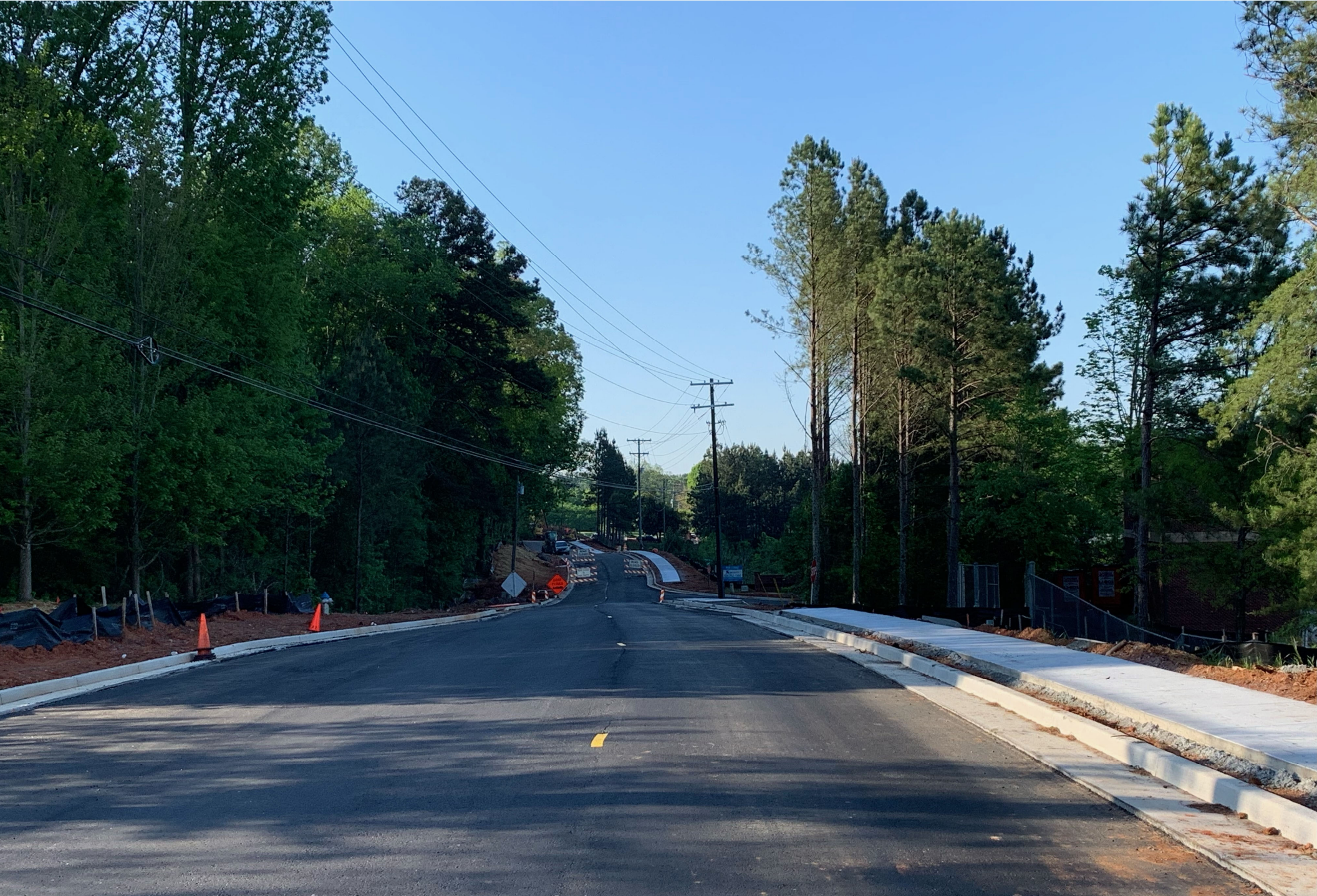
HAMES ROAD RECONSTRUCTION
