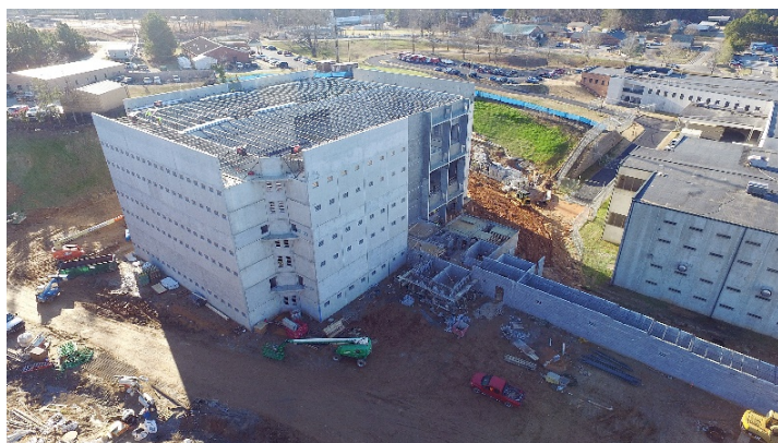
The Adult Detention Center Construction
